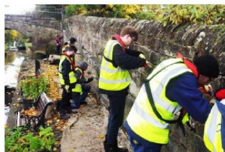
Traditional stonework repairs
